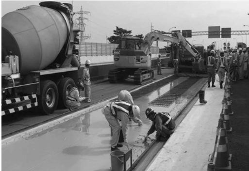
Photo.3 Applying epoxy adhesives
