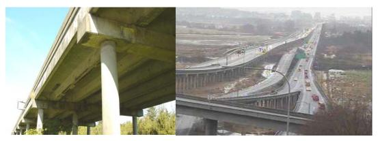
A significant portion of the bridge, 226 spans - 7,410 feet (2259 meters) has conventionally reinforced precast concrete double tee concrete units, also known as inverted tub units. The concrete unit spans approximately 38 feet (11.6 meters) between piers with each span composed of six superstructure units bolted together transversely through their webs.
