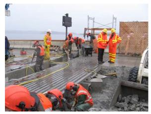
replacement modular joints was greater than that of the originally installed joints. This created some issues with the traffic barriers. When a new bridge is constructed, blockouts are formed in the concrete deck or edge beam to accommodate the modular expansion joint later on. After the modular joint is installed, the concrete barriers are constructed up to the outside limits of the modular joint with steel embedment for attaching steel sliding cover plates.
