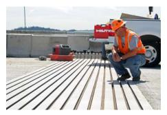
The next technical issue was the gap to set the replacement modular expansion joint in place. The cumulative gap setting is primarily a function of wind and wave motion and water level, not the temperature of the bridge, the floating portion of which is moderated by the temperature of the lake water. It was decided to set reference pins in the roadway slab prior to removal of the existing joints, then to install the
