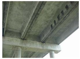
CFRP repaired concrete areas have been inspected with the longitudinal joint repairs and carbon fiber reinforcement performing as originally designed with no visible deterioration. It is anticipated that this repair will provide 25 years or more of service.
