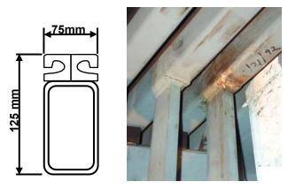
dynamic wheel loads. The location and extent of the cracks were also carefully monitored. Repairs were made in several instances by welding the cracks but nearly all of these locations cracked again.
