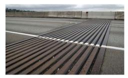
The section of the bridge with the three westbound lanes has two large movement modular joints (48 inch, 122 cm) that are 63 feet ((19.2 meters) in length and the section with two reversible lanes has two large movement modular joints (48 inch, 122 cm) that are 40 feet (12.2 meters) in length. Thus there are a total of four of these sizes of joints
