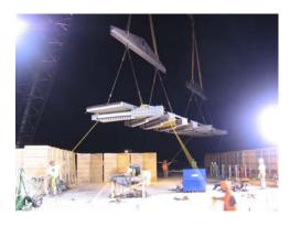
Our Special Provisions required that the contractor submit structural analyses verifying the load carrying capacity of the bridge for the specific cranes that would be used. Given the weight of each joint being installed and the boom radii that would be required to position these joints in their respective blockouts, we realized that the contractor would need some pretty substantial lifting equipment. Additionally, we required that the contractor operate all cranes on a
