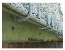
Carbon fiber ply application plans specifying carbon fiber ply tensile capacity requirements were developed for each span for the contract documents. Multiple longitudinal plies where required by the design calculations. In areas where very severe spalling had occurred, transversely oriented carbon fiber plies were specified to resist horizontal shear across the existing concrete-to-repair mortar interface.
