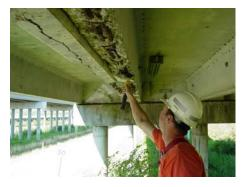
WSDOT contracted with Construction Technology Laboratories to analyze several randomly obtained core samples with the objective of evaluating the technical feasibility of repairing this structure. An analysis of the concrete core samples determined that structural rehabilitation was feasible.
