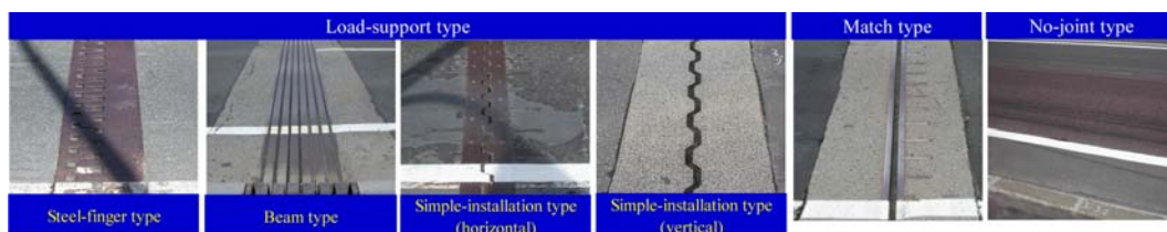
FIG. 1.3 TYPES OF EXPANSION DEVICE
