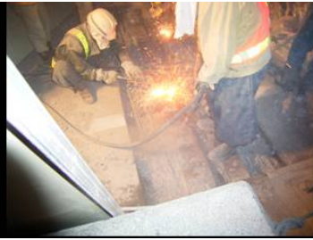
PHOTO 4.4 REMOVAL OF EXISTING DEVICE
