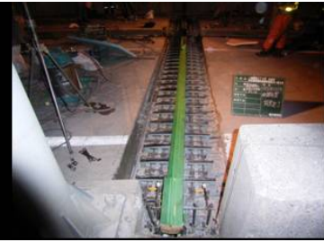
PHOTO 4.5 INSTALLATION OF NEW DEVICE
