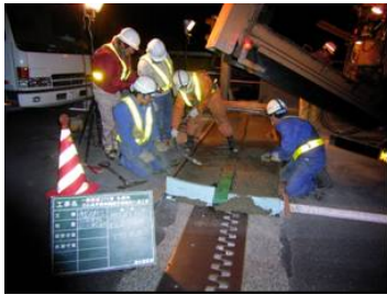
PHOTO 4.6 CONCRETE PLACEMENT
