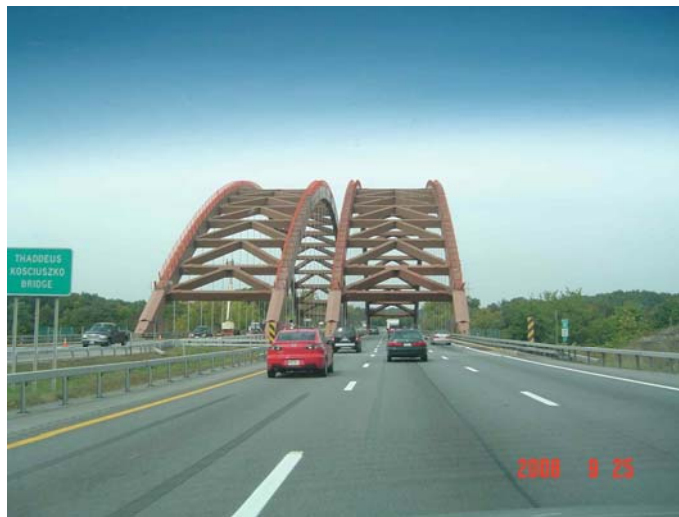
Figure 1 – Northway Twin Arch Bridges (Thaddeus Kosciuszko Bridge), Albany, NY
