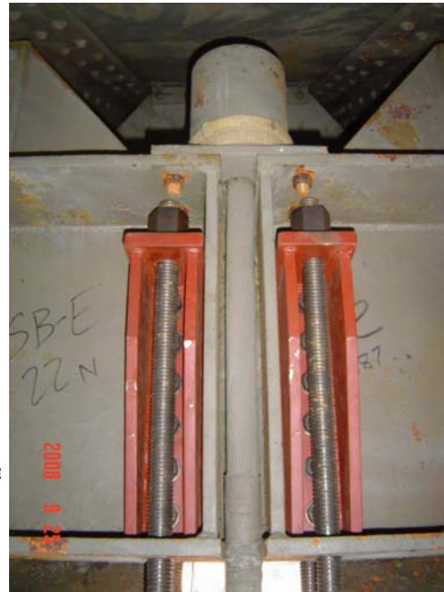
Figure 6 – Connection at Transverse Beam Inside Arch Box
