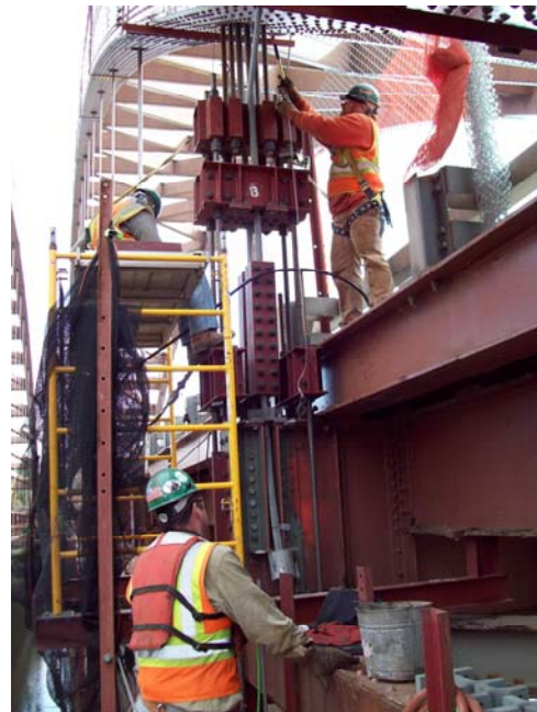
Figure 7 – Structural Lift System Installed at Panel Point 3
