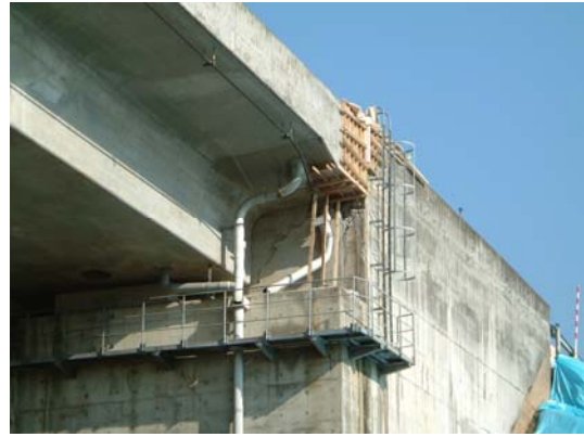
(b) View around girder end
