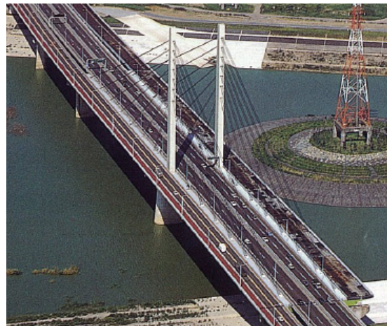
Fig.2 Photo of Sakitama Bridge
