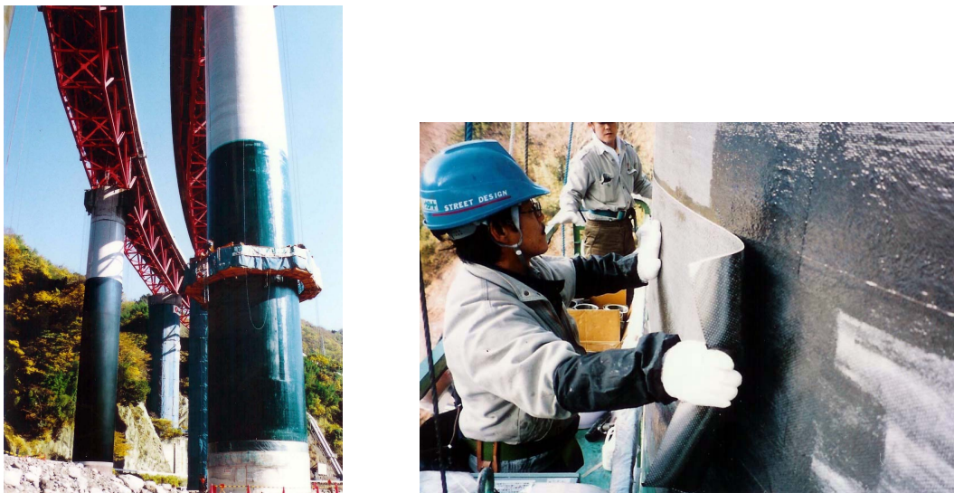
Fig. 1 Retrofit of RC bridge columns with CFRP sheet
