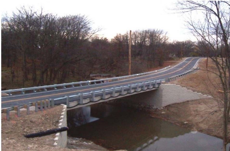
Figure 3 – A recently constructed GRS-IBS bridge
