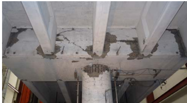
Iowa State University Inverted ‘T’ Bent Cap Testing
