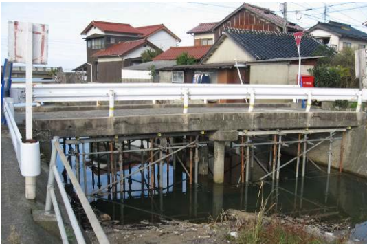
Photo 9 RC Slab Bridge Before Demolition
