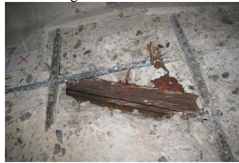
Photo 6 Corroded PC Cables in T-Shape Girder Bridge
