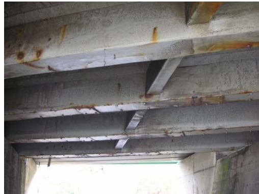
Photo 10 RC T-Shaped Girder Bridge with Multiple Repair Works
