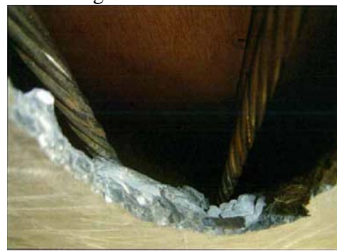
Photo 6 Corroded PC Cables in T-Shape Girder Bridge
