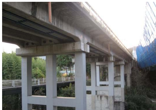
Photo 11 RC T-Shaped Girder Bridge Served about 80 Years
