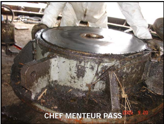
Figure 11– Removal and Reconditioning of the Pivot Bearing
