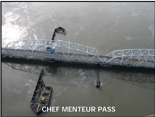
Figure 15 – Pier Protection Systems
