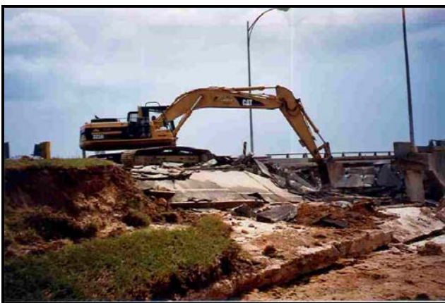
Figure 7 – Abutment and Approach Slab Repair
