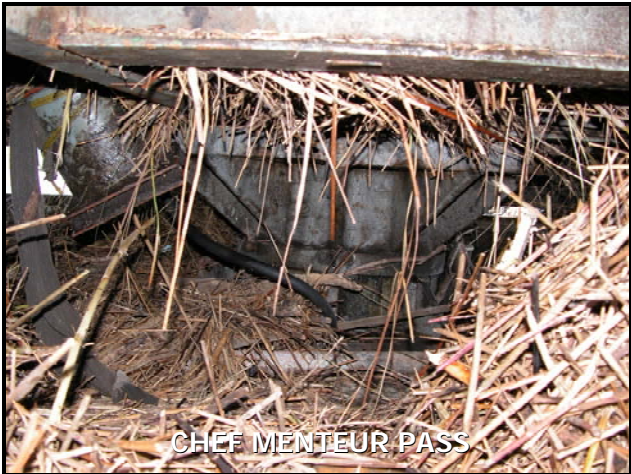
Figure 10 – Inundation of Swing Span Bridges
