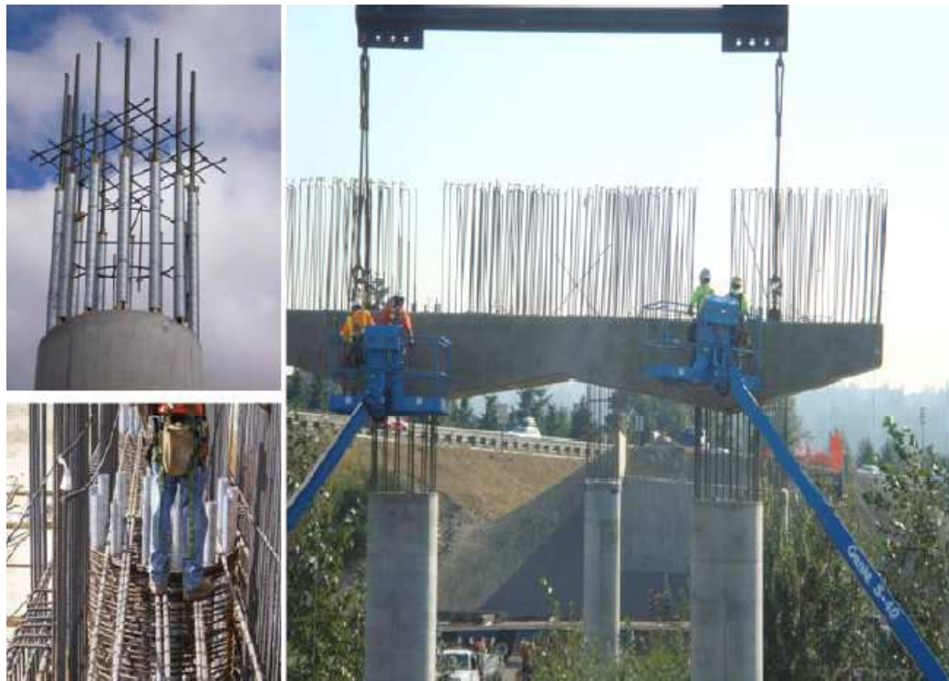
Fig. 4: Precast Bent Cap under construction in Washington State
