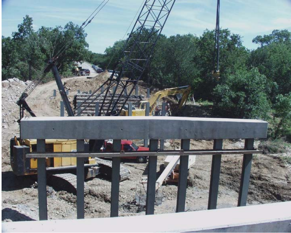
Figure 1, Trestle bent with precast cap on steel H piles
