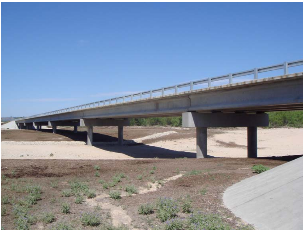
Figure 7, Completed Live Oak Creek Bridge
