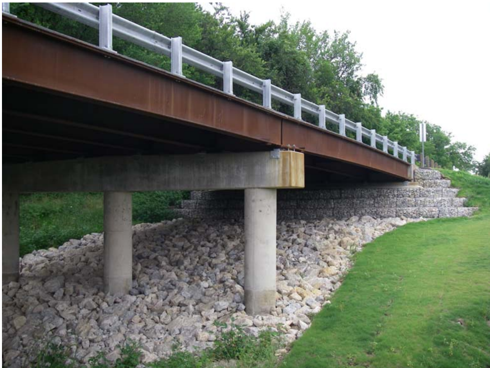
Figure 8, Completed Martin Branch Bridge
