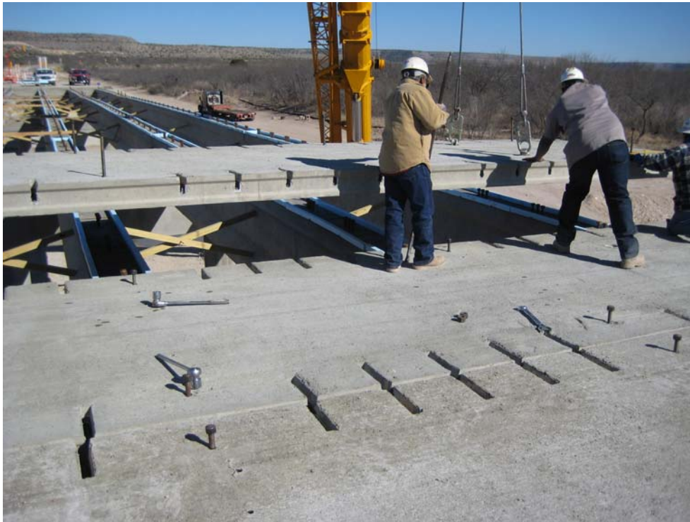
Figure 6, Erection of Full depth deck panels, Live Oak Creek Bridge
