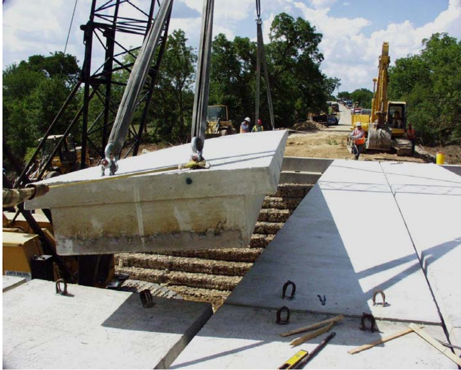
Figure 5, Decked slab beam erection, Salt Creek Bridge
