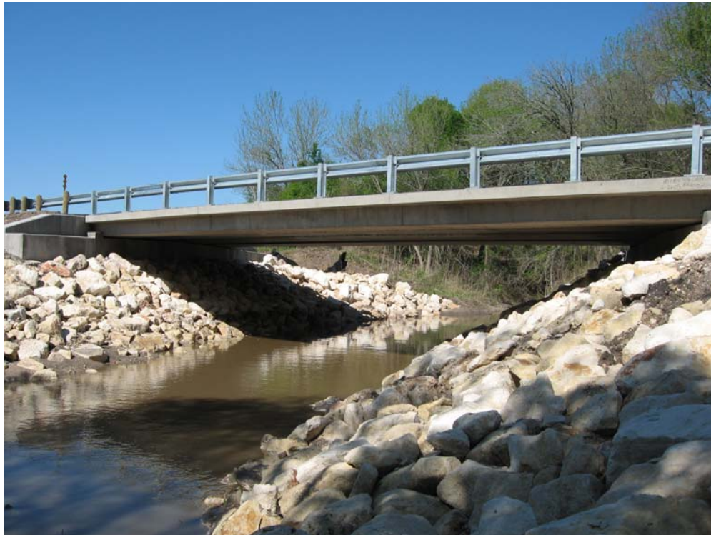
Figure 4, Decked slab beams, Battleground Creek Bridge
