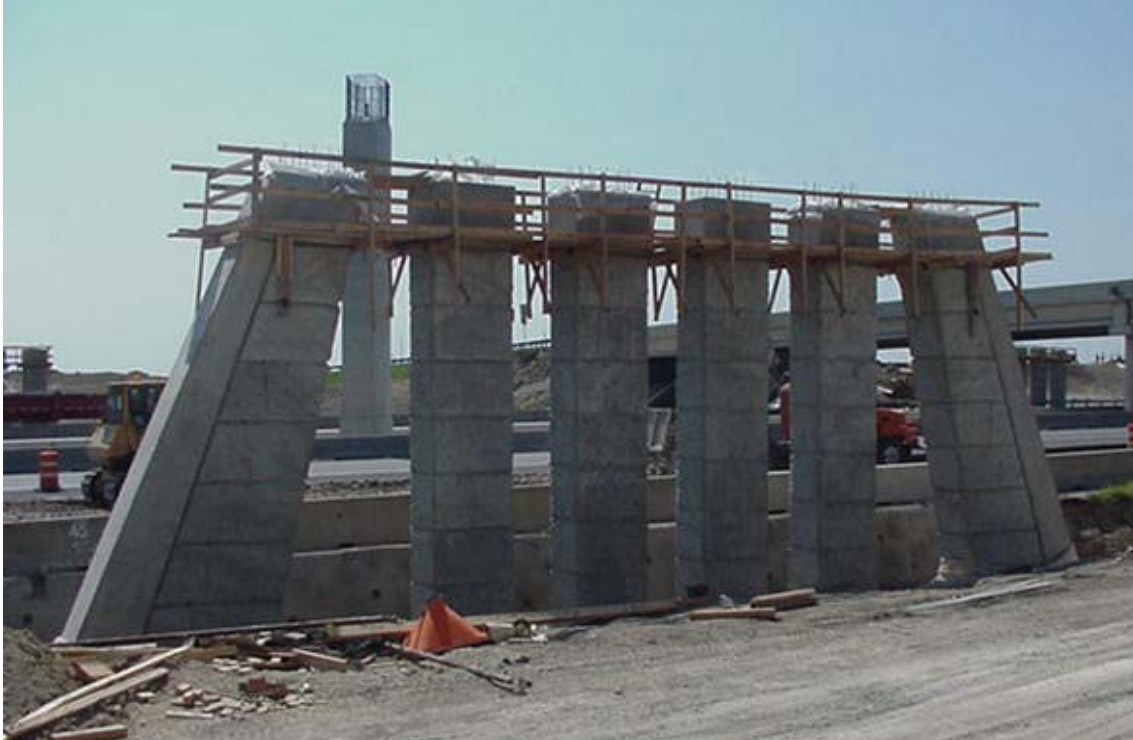
Figure 2, Precast column shells, Loop 340 Overpasses
