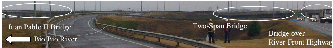
FIG. 12 NE APPROACHES TO THE JUAN PABLO II BRIDGE
