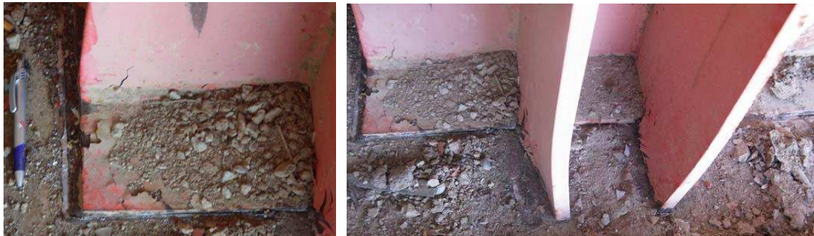
(a) The girder end
