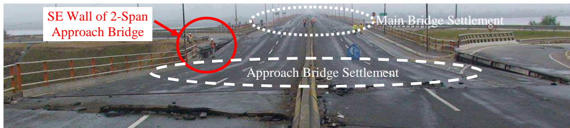
(a) Overall settlement of the Juan Pablo II Bridge (facing the Bio Bio River)
