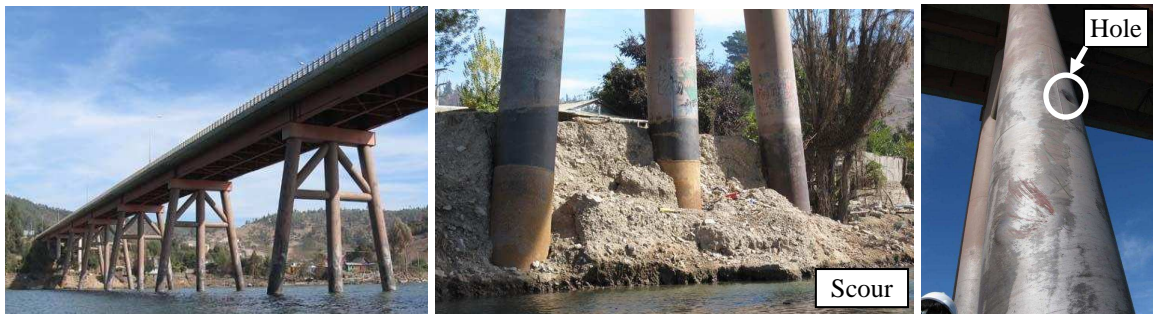
(a) Southern spans and pile bents (b) Erosion of alluvial materials (c) Debris-impact hole FIG. 9 DAMAGE TO THE CARDENAL RAÚL HENRÍQUEZ BRIDGE (MOP)
