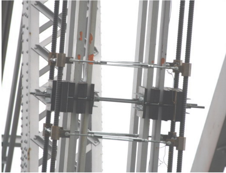
FIGURE 4-DAMPERS ARE DESIGNED TO REDUCE VIBRATION.
