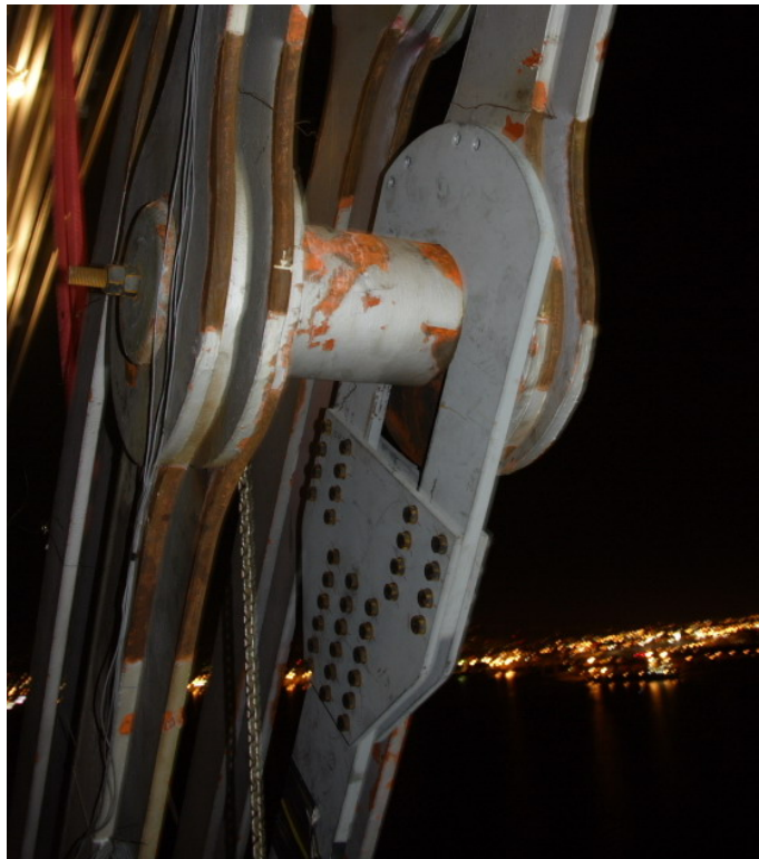
FIGURE 5-COMPLETED REPAIR OF THE PERMANENT EYE BAR.
