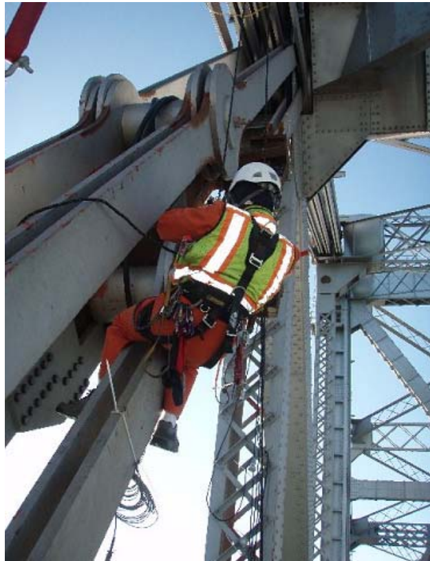
FIGURE 2-CLOSE-UP INSPECTION OF THE DIAGONAL EYE BAR WAS CONDUCTED.
