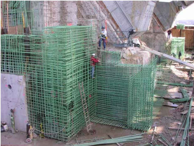
Figure 9. Construction of the encasement
