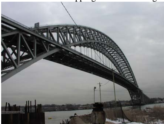
Figure 1. Bayonne main arch span looking south toward Staten Island
