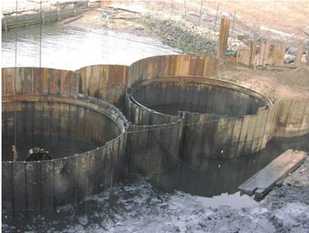
Figure 8. Cofferdam cells during construction
