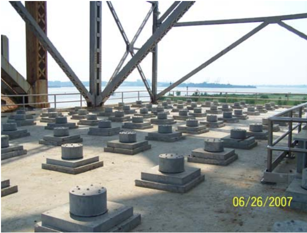
Figure 10. Photo of the top of the abutment after completion of work
