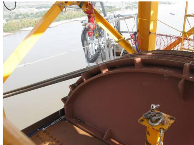
FIGURE 12- TEMPORARY CABLE SUPPORT AT DECK FIGURE 13- TEMPORARY CABLE SUPPORT AT TOWER
