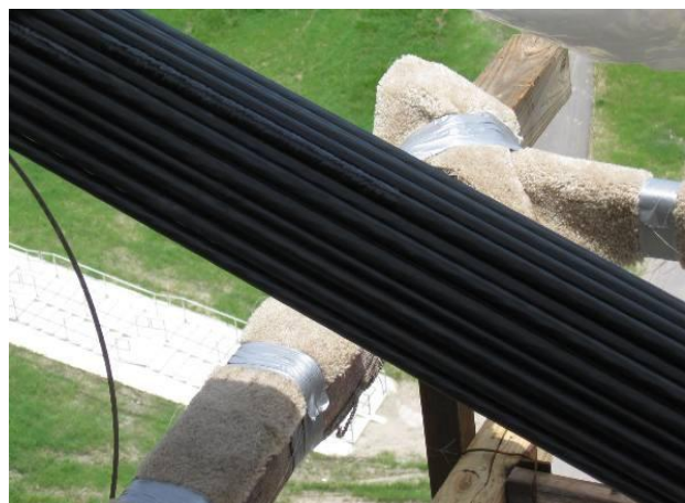
FIGURE 11- STRAND BUNDLE IN A NEW CABLE
