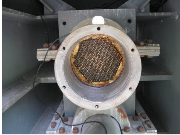
FIGURE 3- AN EXISTING ANCHORAGE SOCKET
