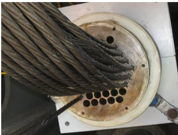
FIGURE 10- A NEW CABLE ANCHORAGE
