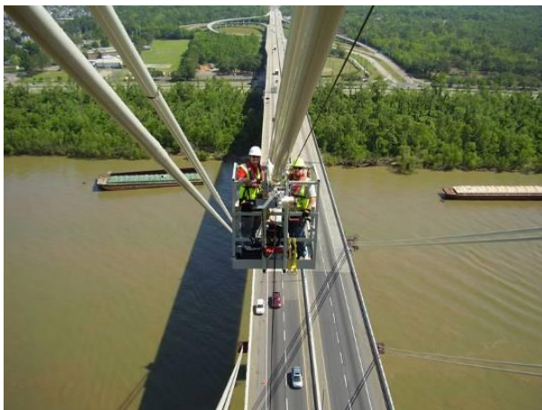
FIGURE 4- INSPECTION ALONG CABLE FREE LENGTH
