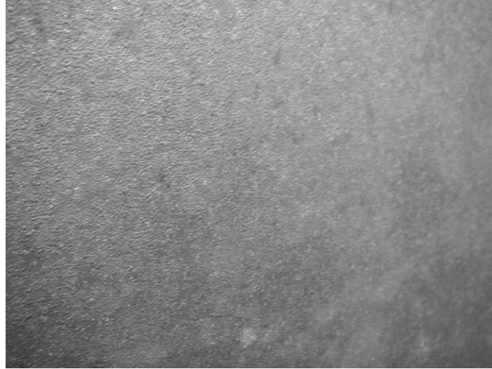
Fig-8 Surface condition at Misaki viaduct
