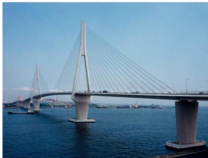
Fig.2 Complete view of the Tsurumi-tsubasa Bridge
