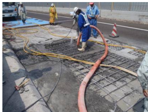
Fig.11 Removing the surface of RC decks with water jet
