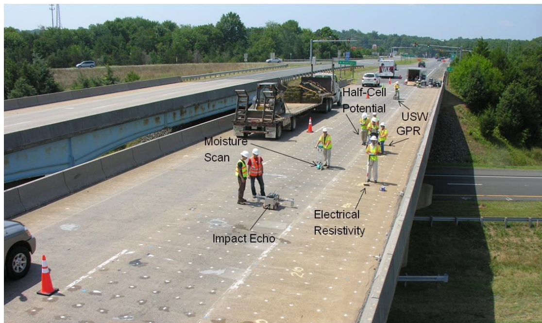
Figure 1. Condition surveys of a bridge deck using multiple NDE technologies.
