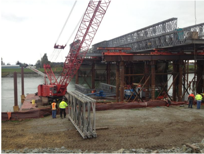
Figure 11: Dismantling of Temporary Bridge on Flexifloat Barge and Removal of piling
