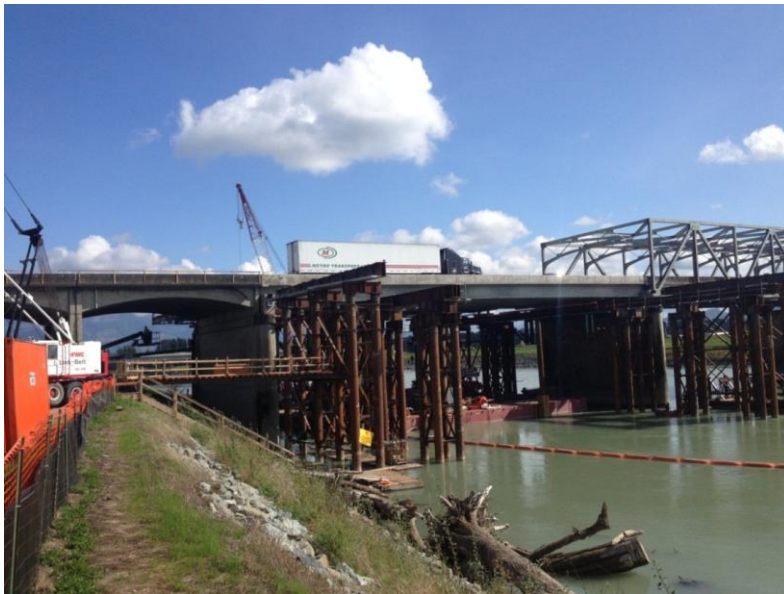
Figure 10: Completion of Span Replacement
