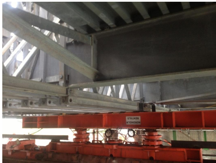
Figure 8: Jacking system for Bridge Slide
