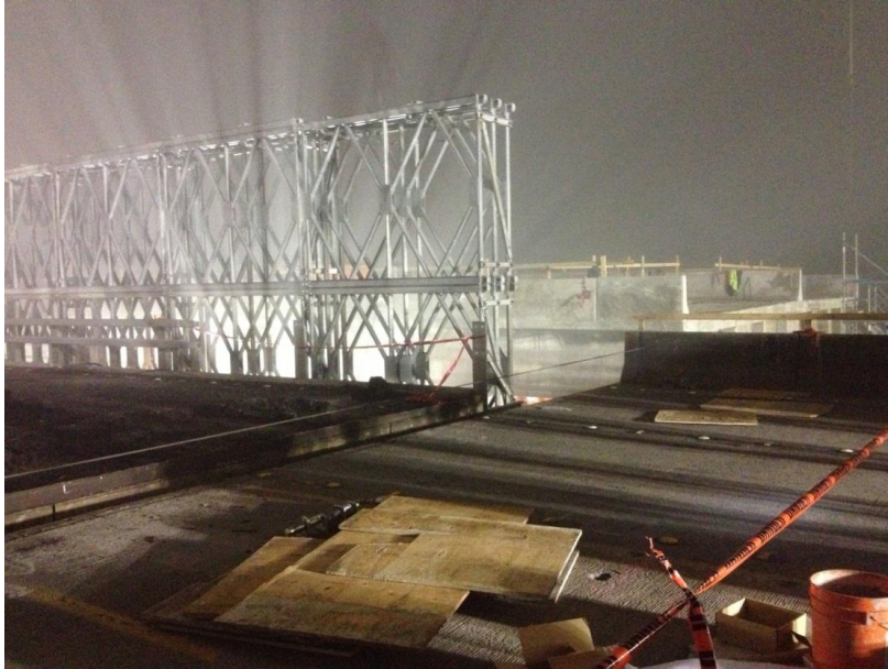
Figure 9: Temporary Bridge Being Slide Out
