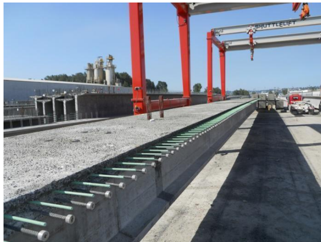
Figure 3: Headed bars at closures
