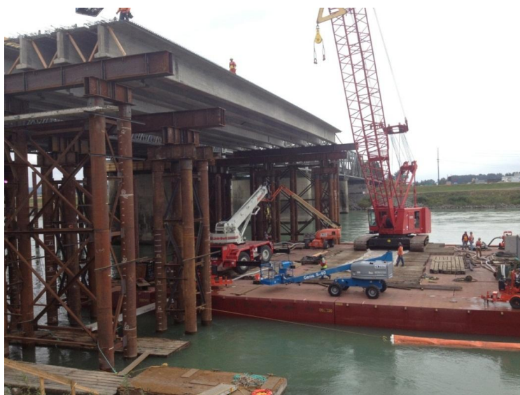
Figure 6: Supports for slide of the new span into place
