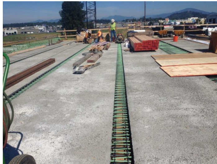
Figure 7: Placement of deck bulb tee girders
