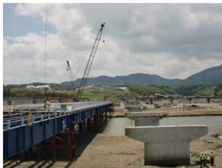
(b) Opened to traffic in 3.5 months of the tsunami strike
