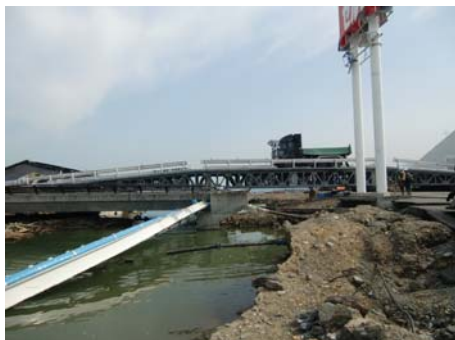
(a) Opened to traffic in 14 days of the tsunami strike
