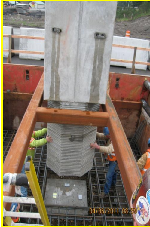
Fig. 5 – Precast column embedded in cast-in-place footing in the State of Washington
