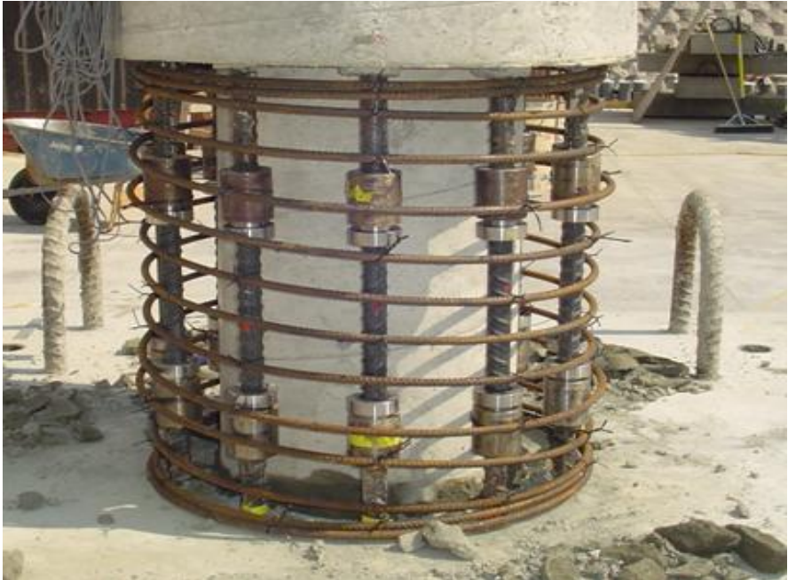
Fig. 7 – Precast column-footing connection model with headed bar couplers tested at the University of Nevada - Reno
