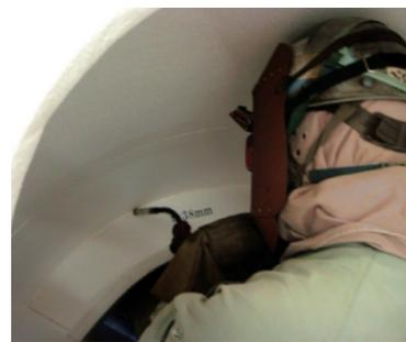
(b) Situation for checking the quality of welding workability using full scale model.
