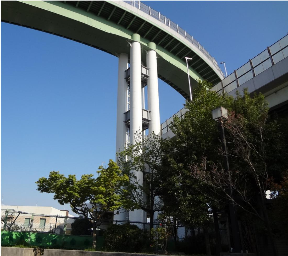
**Picture-5 Steel Pipe Integrated Pier with Shear Link (Ebie junction)**
