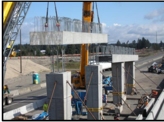
Figure 3. Construction of Precast Column Bent (without pretensioning)
