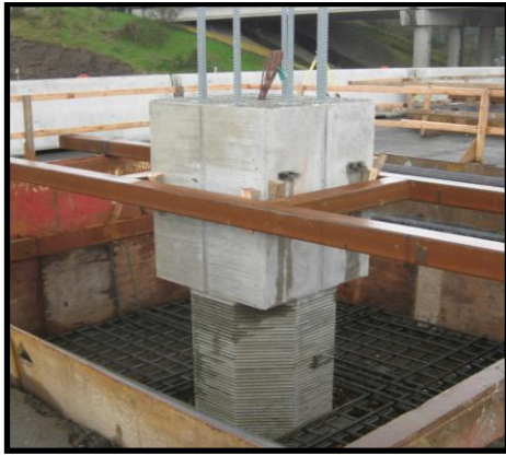
Figure 3. Construction of Precast Column Bent (without pretensioning)
