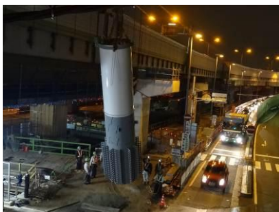
Photo-3 Erecting steel pier
