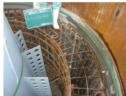
Photo-4 Inside the socket steel pipe
