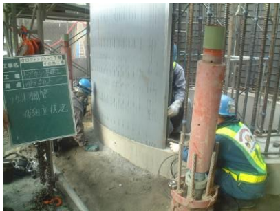
Photo-1 Erecting socket steel pipe
