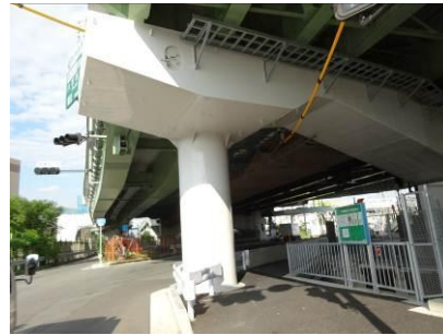
Photo-6 Finished construction
