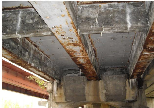
Photo 1 Steel plates bonded to the soffit of girders in a concrete bridge
