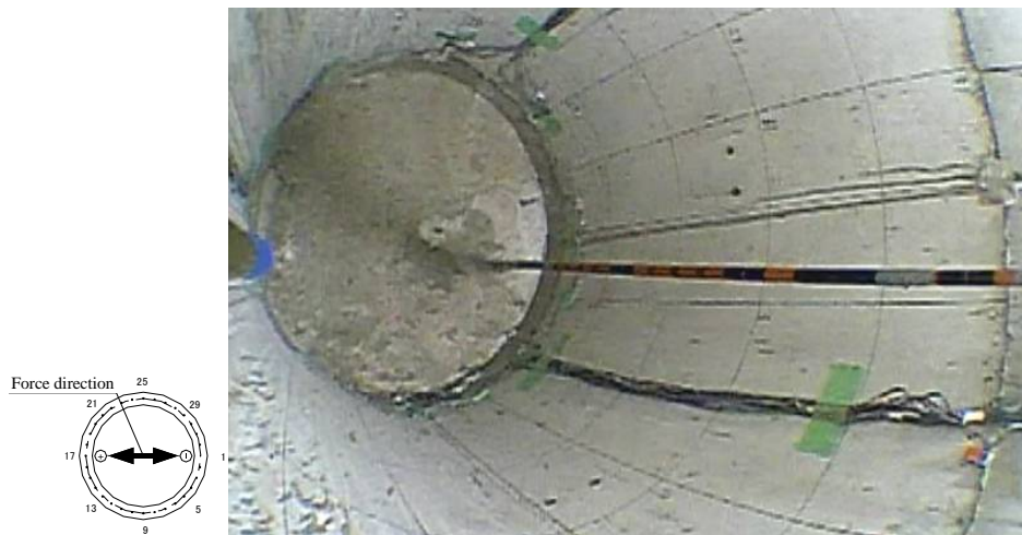
(b) Damage observed at inside face
