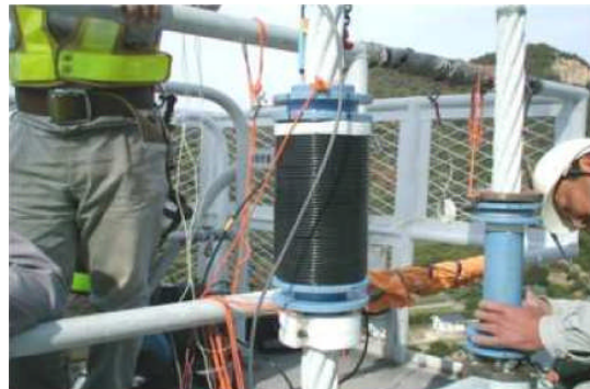
Photo 5 Application of Main Flux Method
