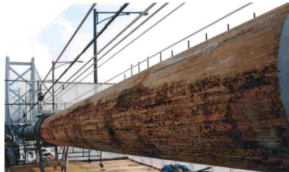
Photo 2 Unwrapped Main Cable of Kita Bisan-Seto Bridge
