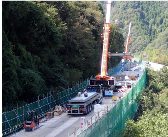
Pic. 2 Construction status during road closure
