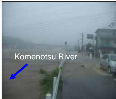
Overflowing in the upper reach of Hirosebash Bridge
