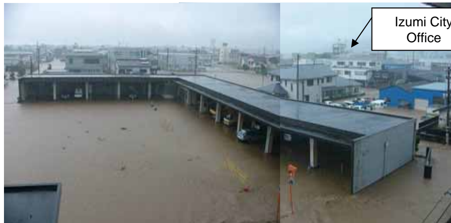
Inundation in right side of Komenotsu River
