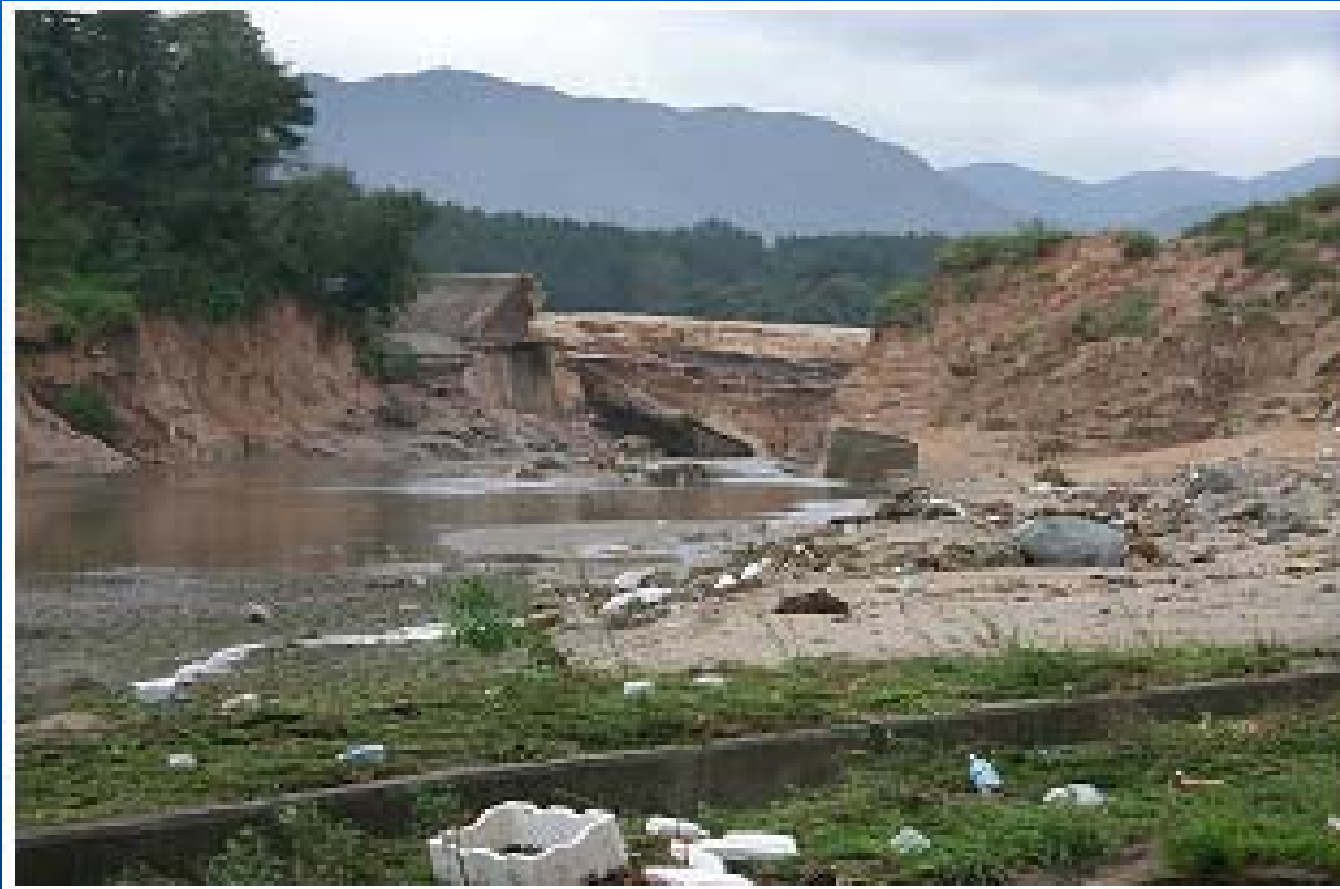
Destroyed Spillway (Gangneung-si, Gangwon-do)
