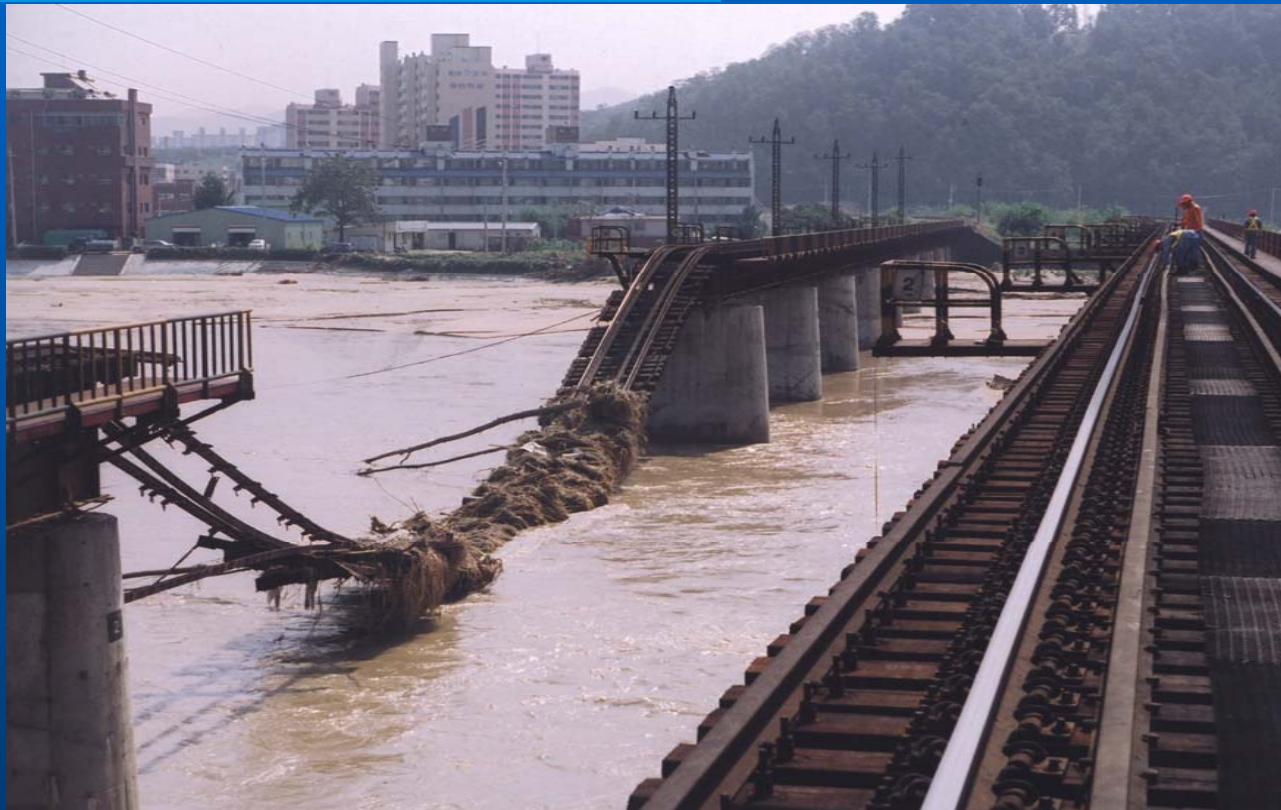
Broken Gamcheon Railway Bridge (Gimcheon-si, Kyeongsangbuk-do)
