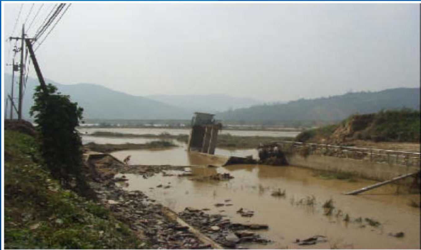
Broken Hoecheonje Levee (Goryeong-gun Gyeongsangbuk-do)
