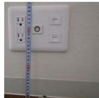
Electric outlet and modular jack with slots 20cm from floor
