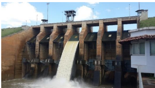
Figure 2: Normal spillway and emergency spillway of the BPL (view from downstream)
