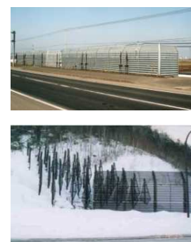
図-5 防雪柵の端部対策例
