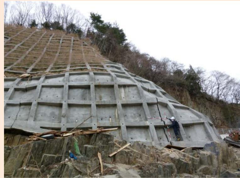
Cracks along joints of crib works (Kawajiri area)
