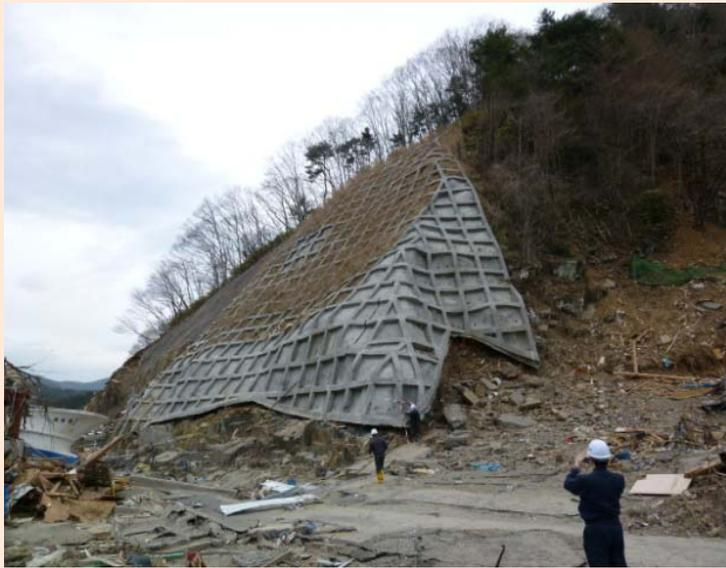
Loss of foundation ground of crib works (Kawajiri area)
