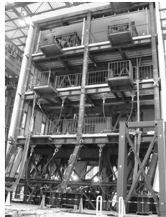
E-Defense Steel Collapse
