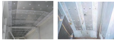
Steel plate bonded
