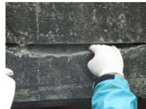
④ 補修材充填
