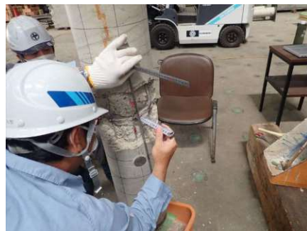
(b) 剥離深さの計測状況
