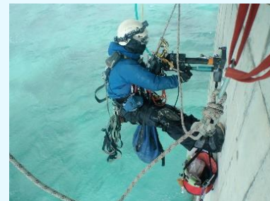
Coring analysis is performed regularly in collaboration with the road administrators
