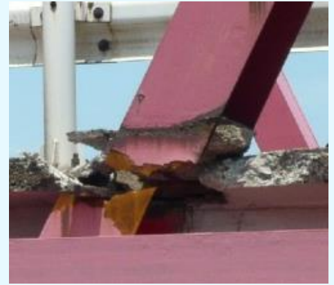
Fracture of the truss member of Kisogawa-ohashi Bridge
