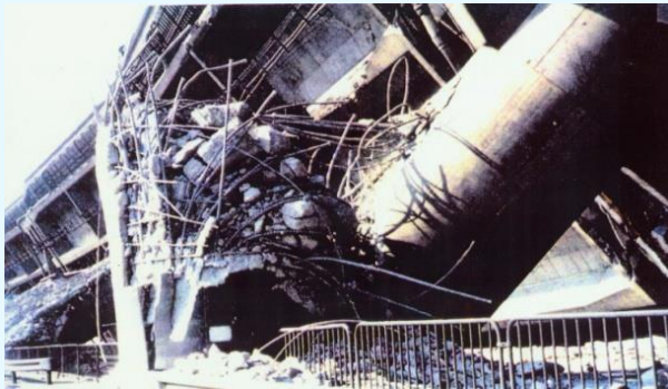
Collapse of a highway viaduct of Route 3, Kobe route, of the Hanshin Expressway during the 1995 Hyogo-ken Nanbu Earthquake
