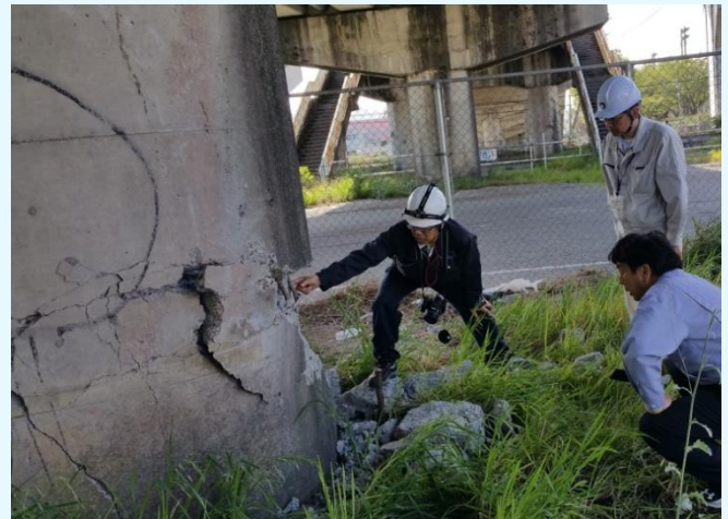
Damage examination of road bridges following the Kumamoto earthquake
