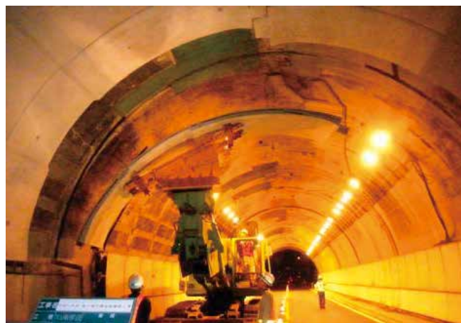
Application example of tunnel inner reinforcement
