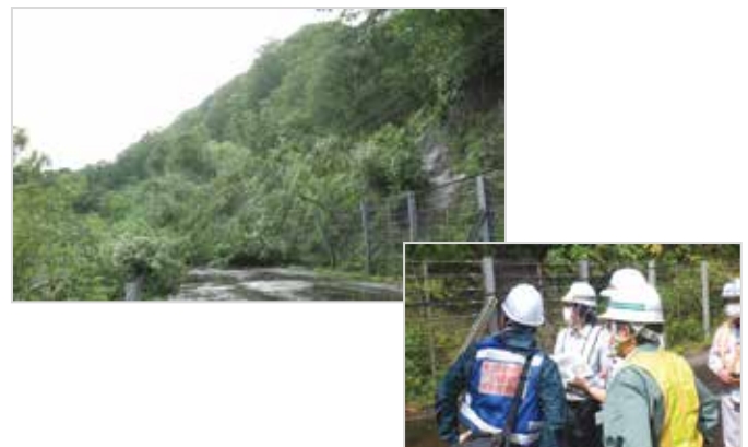
August 2022 slope collapse on National Route 277: On-site investigation of the mechanism of the surface collapse (photographed on August 17, 2022)
