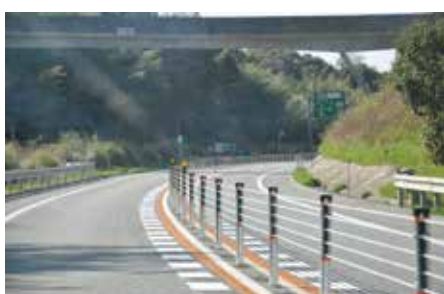
Installation status: Hamada Expressway
