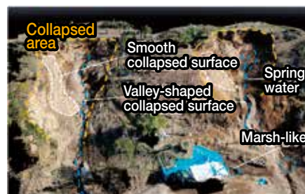
Geomorphic analysis using BIM/CIM to understand the mechanism of collapsing landslides
