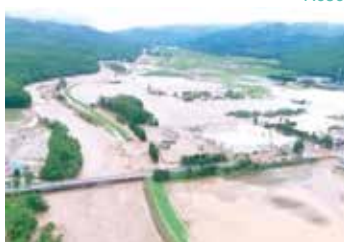
Breaking of the Sorachi River levee in the Ishikari River system
