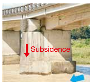
Hydraulic analysis aimed at clarifying the scouring damage mechanism of bridge piers that subsided due to flooding (Riverbed variation around the damaged bridge pier expressed by two-dimensional riverbed variation calculations)
