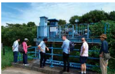
An introduction to the latest research in Japanese river restoration for biodiversity enhancement, presented to visitors from the UK. (Photo: A movable weir inducing flooding in an experimental stream)
