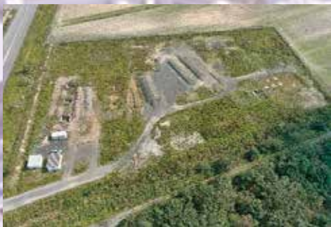
Construction Test Field in Tomakomai (Tomakomai City)
