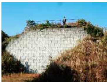
◀ Experimental reinforced soil wall (8 m height) for long-term observation
