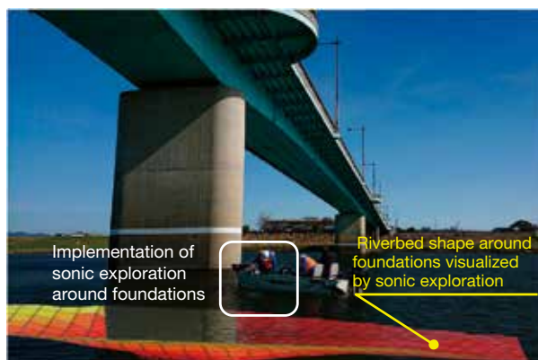
Trial of preventive maintenance technology (underwater visualization technology to determine the state of foundation scouring)
