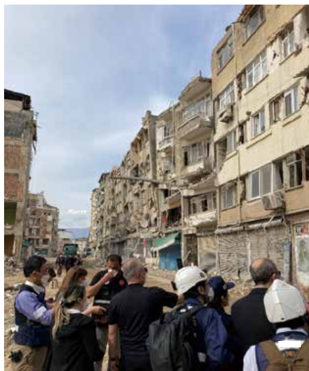
Damage survey of buildings on soft ground (provided by JICA)
