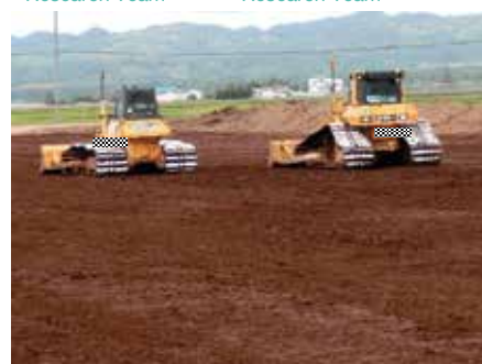
Field in which large-scale partitioning is carried out when the soil moisture is appropriate to prevent the worsening of soil physical properties such as drainage
