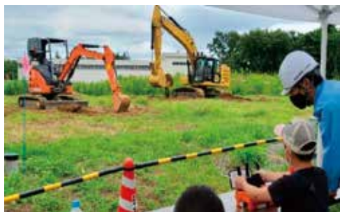
Experience with remote operation technology that allows construction work to be performed safely at dangerous sites
