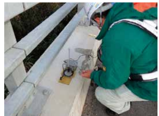
Evaluation of concrete surface quality through surface water absorption tests
