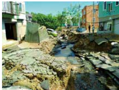
Damage to residential areas due to liquefaction
