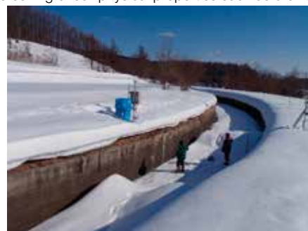
Survey of the deterioration of agricultural open canals caused by freeze-thaw effects unique to cold regions
