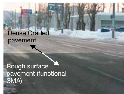
Example of winter road surface measures using rough-surface pavement
