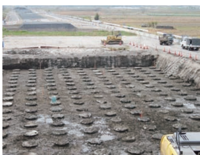
Soil improvement work at Maibara Bypass
