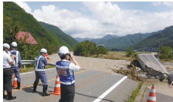
Typhoon No.10 etc.: Field survey of the collapsed bridge in Hidaka Town (1 Sep.)
