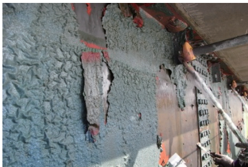
Coating film being peeled off
