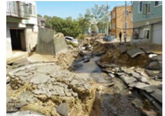
Liquefaction damage in a residential area
