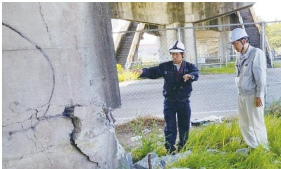
Kumamoto Earthquake: Inspection of damages at the crossover in the City Road Chuo Line (Apr. 17, 2016)
