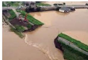
Levee breach by piping
