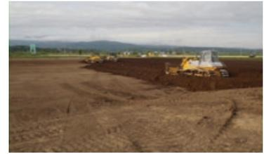
Construction of large-sized paddy field: Decision on selection of machinery and construction timeframe based on the soil diagnosis is required.
