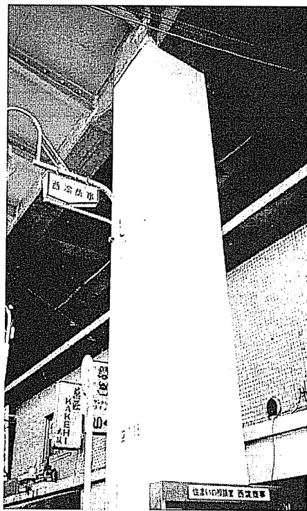
Figure 4 Composite Material (FRP) Wrapping Used in Limited
