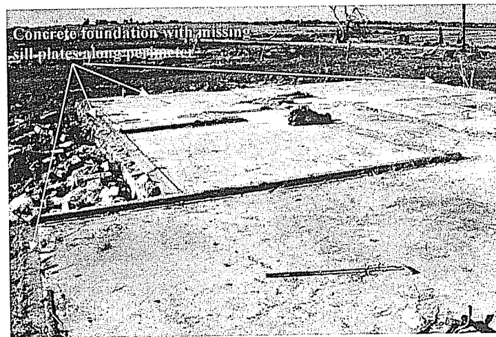
Figure 3. Close-up view of a typical slab-on-grade foundation of houses in Jarrell. Only one sill plate remains connected to the concrete foundation.
