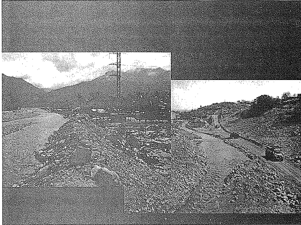
Figure 7: Preparation for Future Flood Protection Through Channel Clearing and Construction
