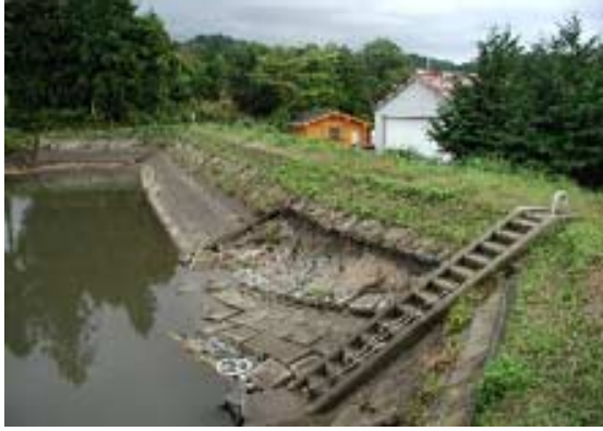
Figure 13 Sliding of upstream slope at Kanayatani Irrigation Dam
