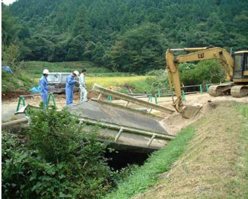
Photo 2 Collapse of girder, Harada bridge, Akantani municipal road of Seihaku town
