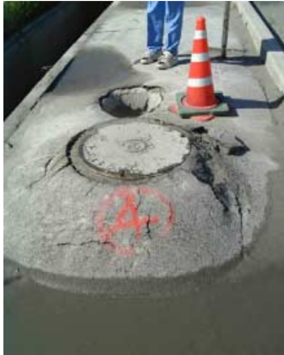
Photo 8 Projection of a sewage treatment manhole, Takenouchi Industry Complex
